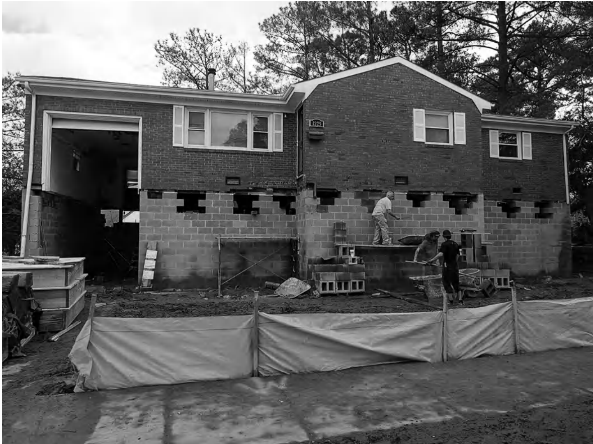
Figure 20.3. Some homeowners have begun raising their homes to prevent flooding.
