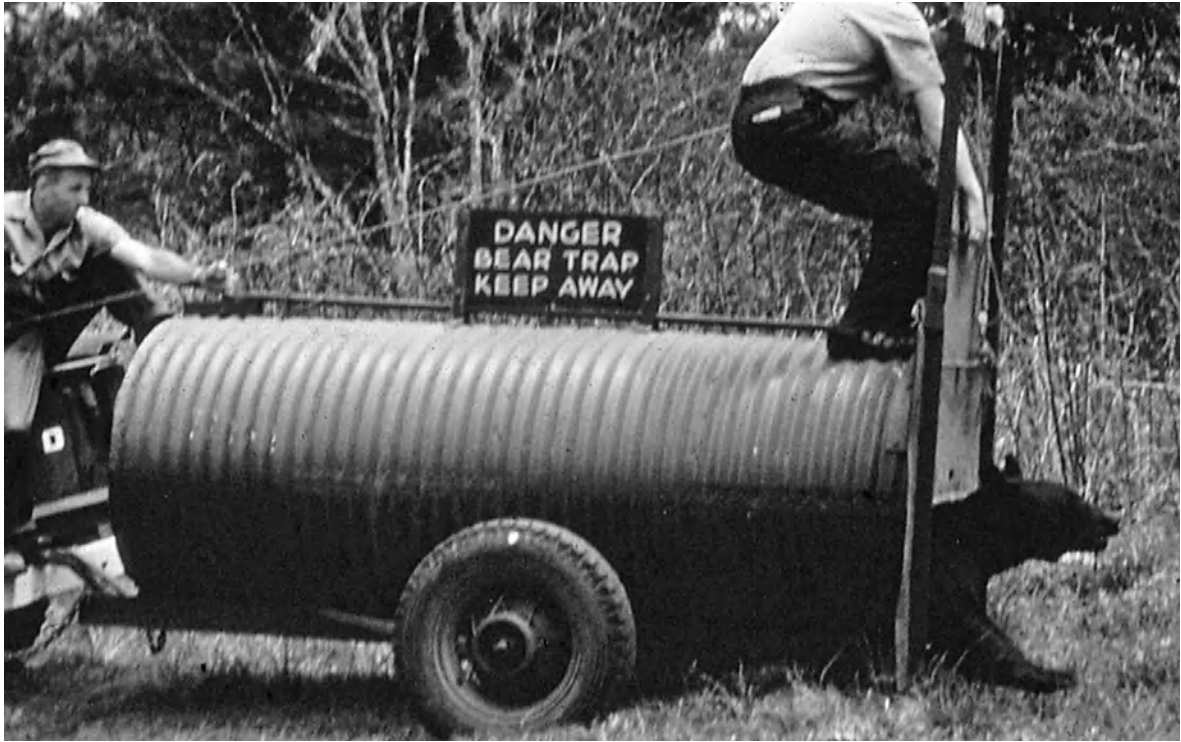
Figure 15.3. Culvert trap used for capturing bears in Great Smoky Mountains National Park.
