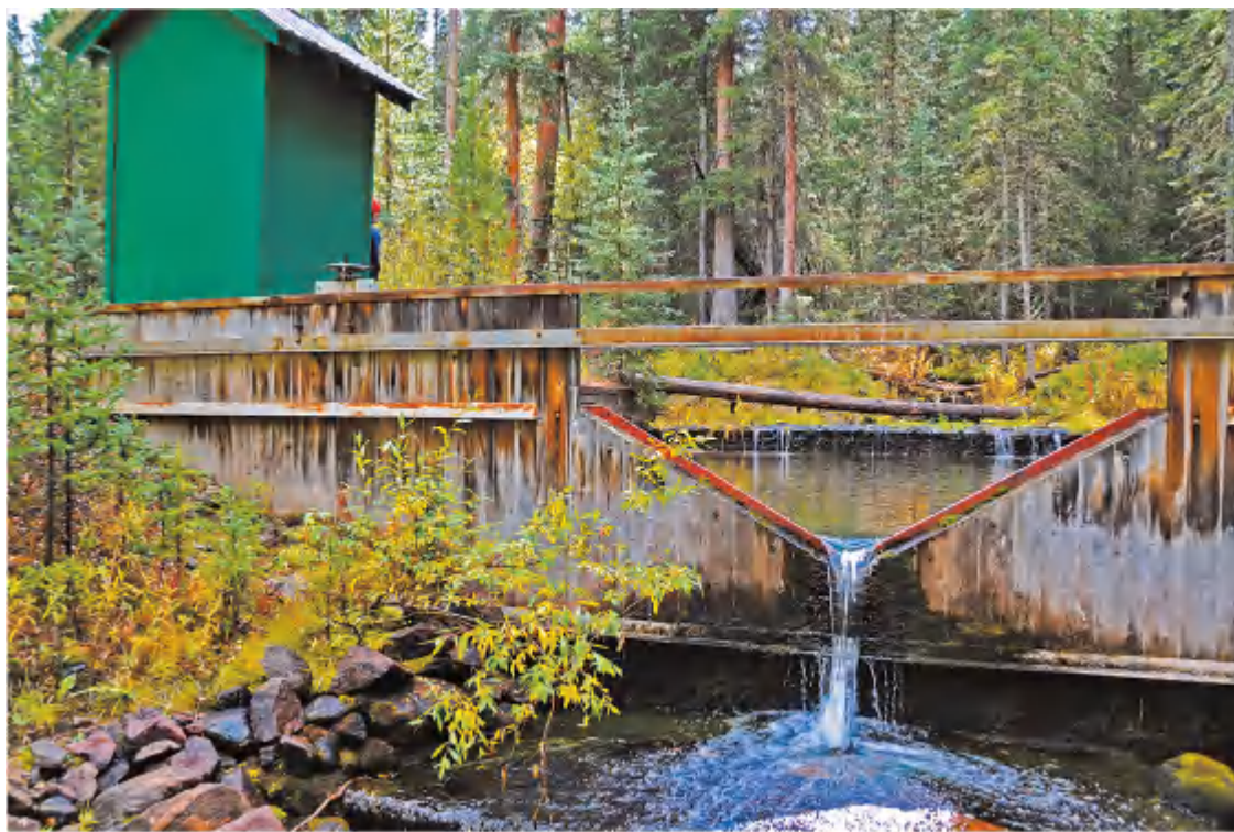
FIGURE B Measuring Water Flow A weir on Fool Creek in the Fraser Experimental Forest, Colorado.
