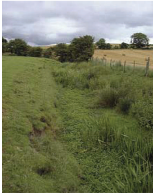
Figure 5 Choked watercourse, River Skerne, UK. Source: P. Widdison.
