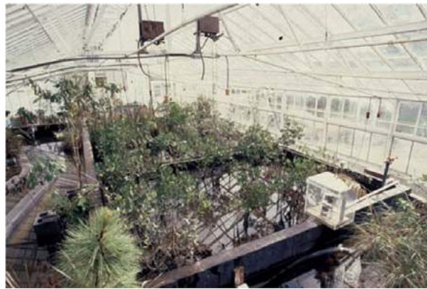
Fig. 1 Florida Everglades mesocosm during construction. The butyl rubber-lined concrete block walls were used to constrain the entire system as well as to physically separate the salinity subcomponents thereby creating a salinity gradient. The plastic box at the lower right contains the tide controller, which determines the tide level in the estuary (center tank and the four smaller units behind).
