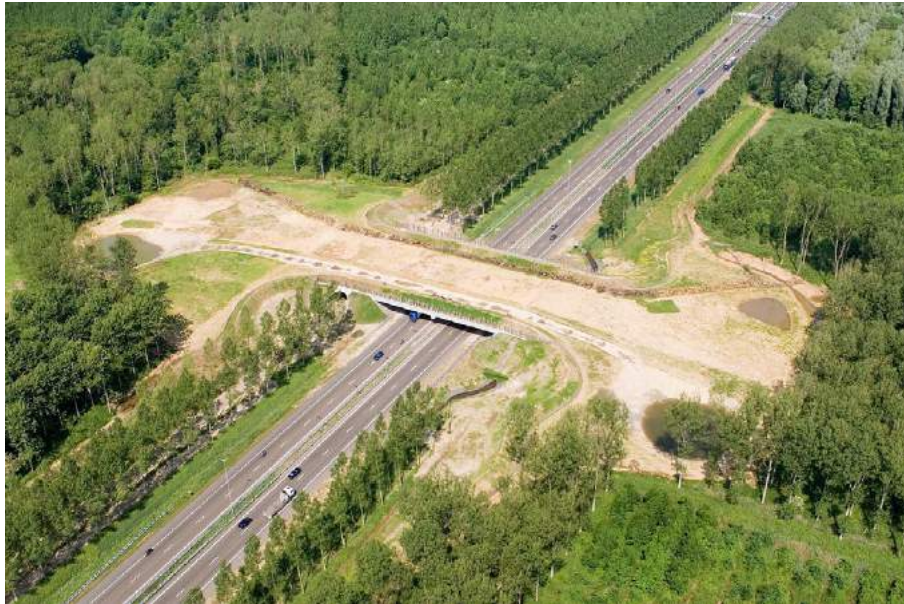
Fig. 6 Ecoduct Groene woud in motorway A2, the Netherlands (photo Rijkswaterstaat).
