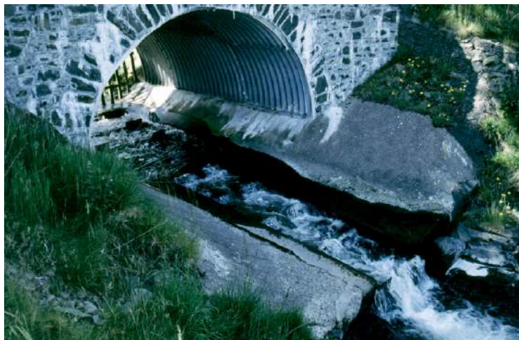
Fig. 9 Fish ladder in one of the headwaters of the Tweed (Scotland) for migration of Salmon ( Salmo salar ) to its spawning waters. (photo Rob Jongman).
