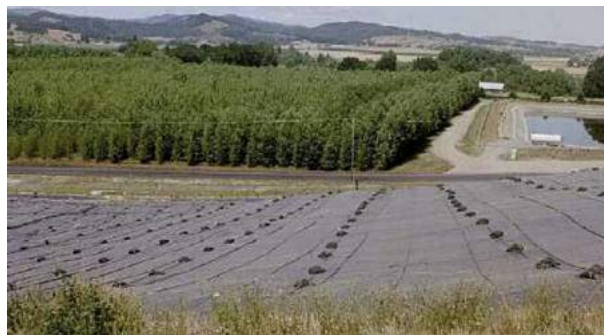
Fig. 5 Eastern Oregon landfill (foreground) leachate collection system (see storage pond on right) and hybrid Populus spp. plantation irrigated with leachate (upper left and center) and harvested for paper and pulp. Originally courtesy of Jim Jordahl, CH2M Hill Consulting Engineers and Scientists, Des Moines, Iowa.
