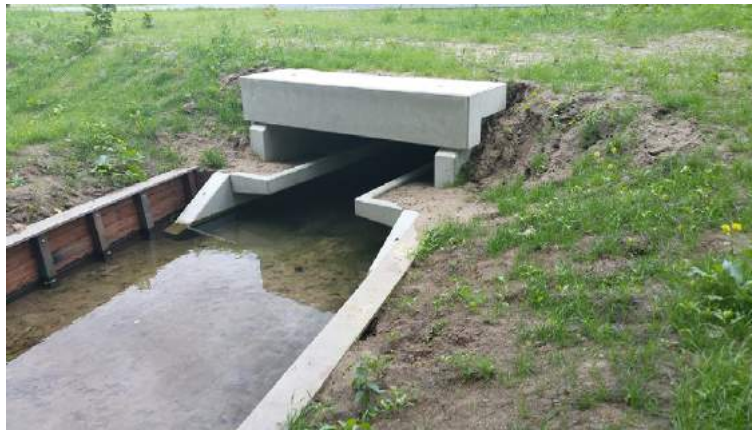
Fig. 8 Adapted culvert as wildlife underpass for small mammals (photo Rob Jongman).
