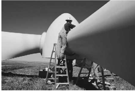
FIGURE 2 Site assembly of large wind turbine nacelles and blades.
