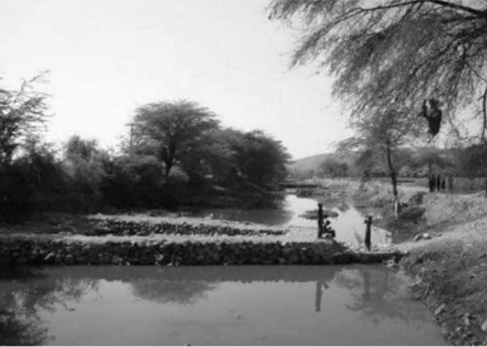
FIGURE 11 Green Bridge installation for ecological restoration of Ahar River of Udaipur, India (courtesy of SERI, Pune, India).
