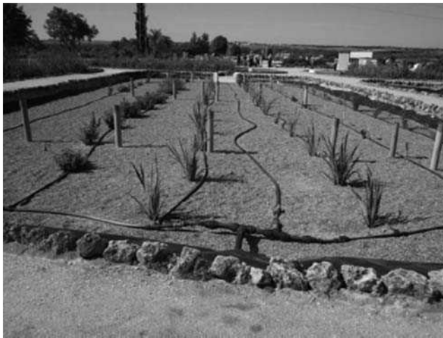
FIGURE 4 Distribution of wastewater on the surface of a vertical flow constructed wetlands. Experimental station, Carrión de los Céspedes, Spain. (Source: Photo courtesy of Jan Vymazal).
