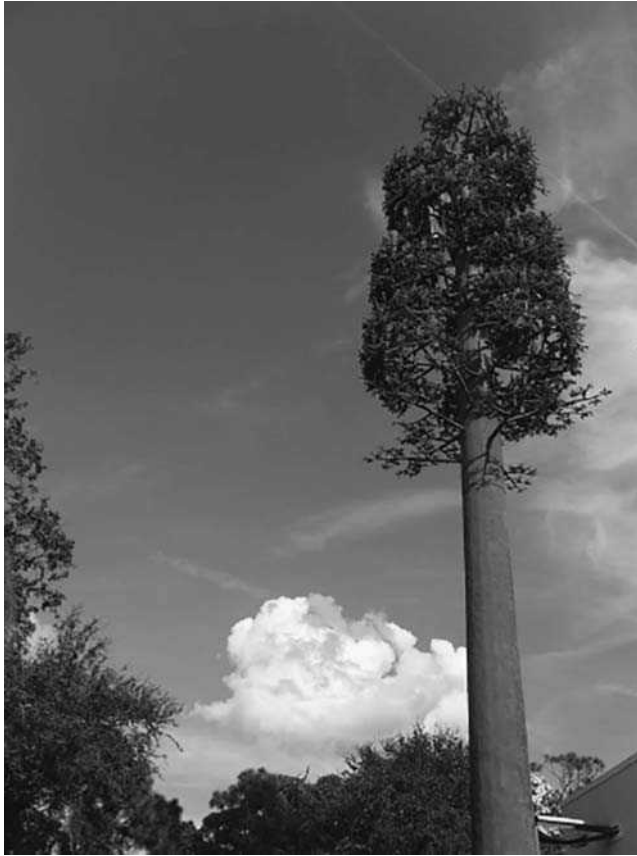
FIGURE 4 RF tower with elaborate camouflage.
