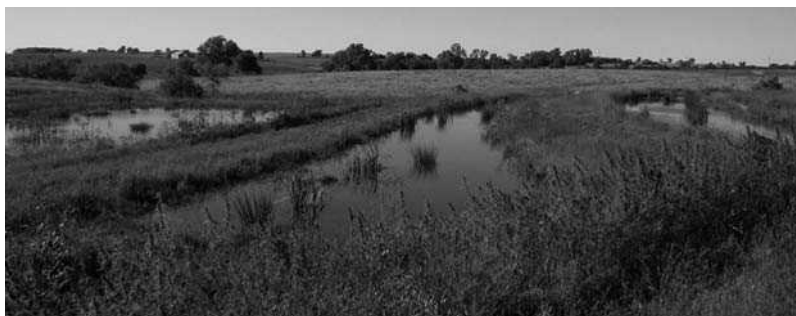
FIGURE 2 A three-cell, FWS wetland for treating dairy wastewater. This system is in its first year of operation; plants were recently established.
