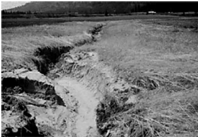
FIGURE 2 Gully erosion from snowmelt runoff in northern Idaho.
