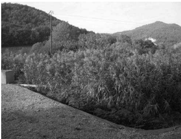
FIGURE 5 Vertical flow CWs at Saint Thomé, France. (Source: Photo courtesy of Jan Vymazal).
