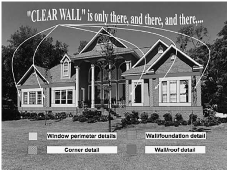
FIGURE 3 Framing lies behind a significant portion of the wall area in many houses.
