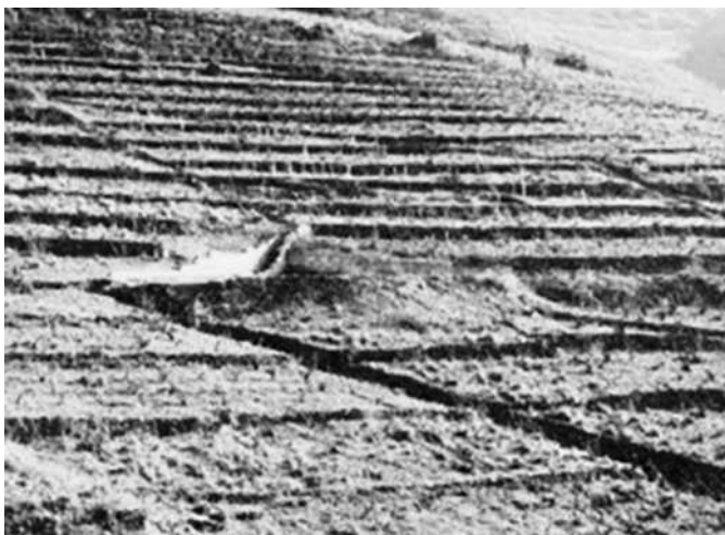
FIGURE 13 Conservation structures showing drop spillway and flumes to convey water downslope, along with stone barriers, in Spain. Source: Reichert and Cassol. [43]
