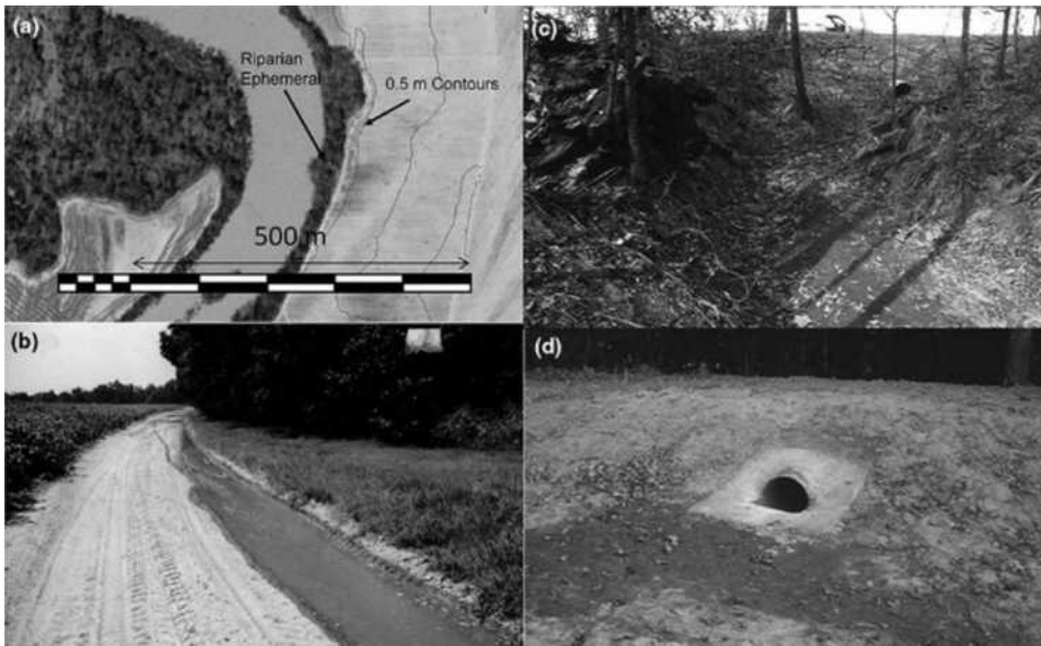
FIGURE 4 Runoff reaching (a) a filter strip/riparian forest buffer surrounding an oxbow lake in the Mississippi Delta was (b) redirected by a small tillage berm to (a and c) a riparian ephemeral flow channel. Storm flow through this channel was controlled by (c and d) a slotted inlet pipe and associated earthen pad, which created backwaters that allowed the riparian buffer to function ( Source: Dabney, Moore, and Locke. [38] )
