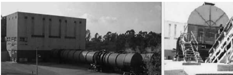
FIGURE 8 Composting rotary drum: (left) side view and (right) view from the waste admission side.
