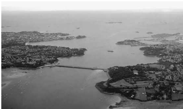
FIGURE 10 Aerial photograph of the world's biggest tidal power station. The Rance Tidal Power Station is located at La Rance (NW France) in the mounding of River Rance, next to the famous island Mont St. Michel.
