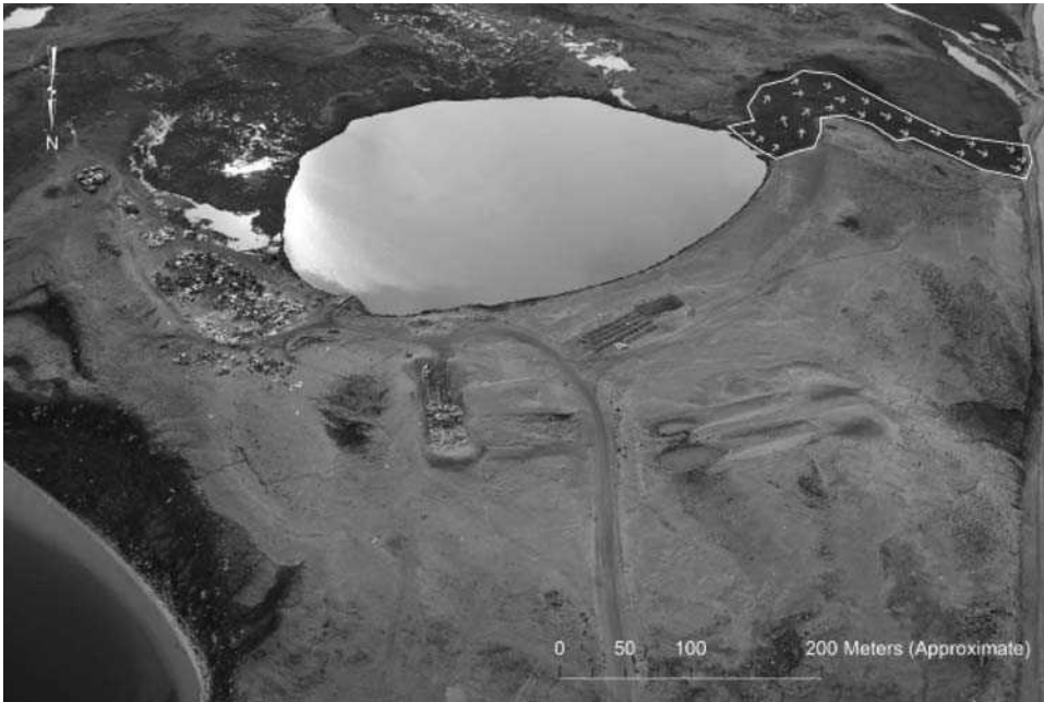
FIGURE 2 Aerial view of Paulatuk facultative lake and treatment wetland. The wetland is located on the upper right of the photo. Effluents flow to the right and a distance of approximately 350 m to the Arctic Ocean. Source: Photo courtesy of Aboriginal Affairs and Northern Development Canada North Mackenzie District.
