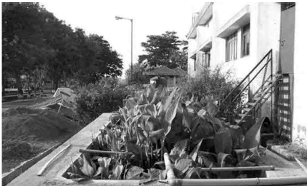
FIGURE 10 Sewage treatment using soil scape filter (courtesy of SERI, Pune, India).
