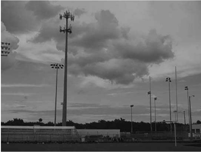
FIGURE 10 RF tower installed adjacent to football field.
