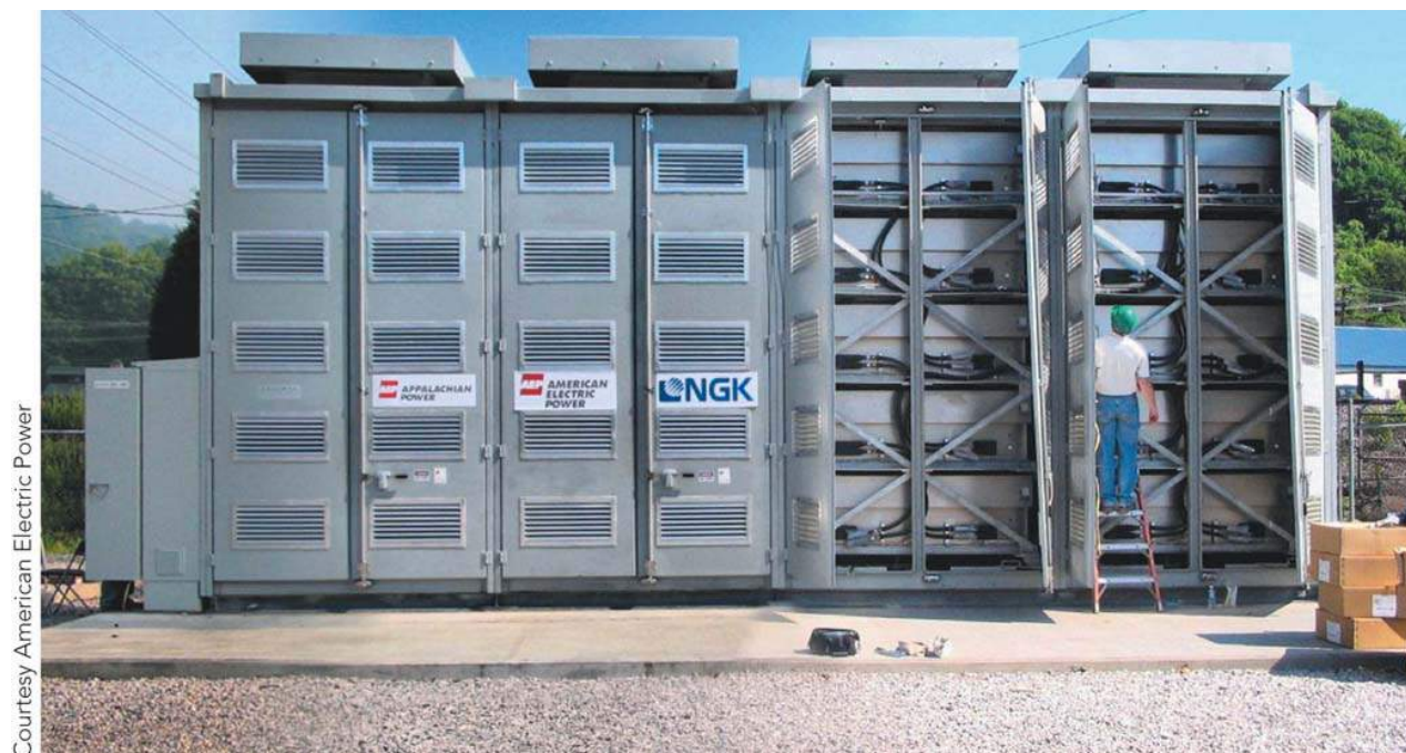
FIGURE 10.11 Sulfur-sodium battery for large-scale energy storage
