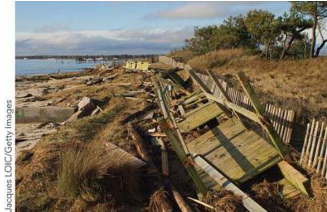
FIGURE 17.17 Storm damage on a coastal dune
