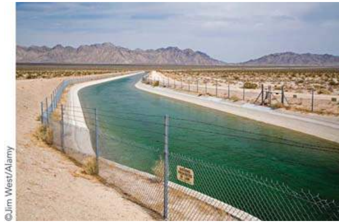
FIGURE 13.12 An aqueduct in California's Mojave Desert
