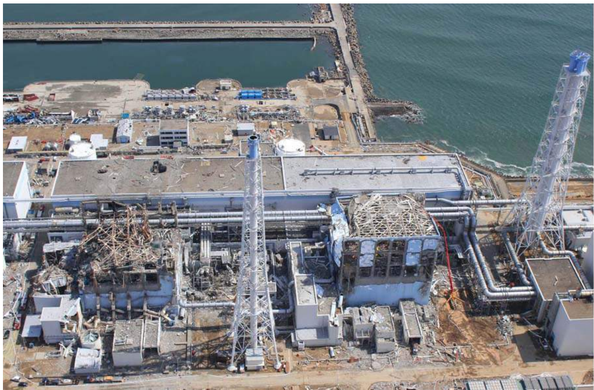
FIGURE 12.18 Damaged Fukushima Daiichi Nuclear Power Plant
