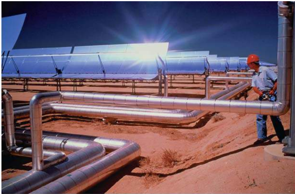
(a) A solar thermal plant in California uses troughs to focus sunlight on a fluid-filled tube.
