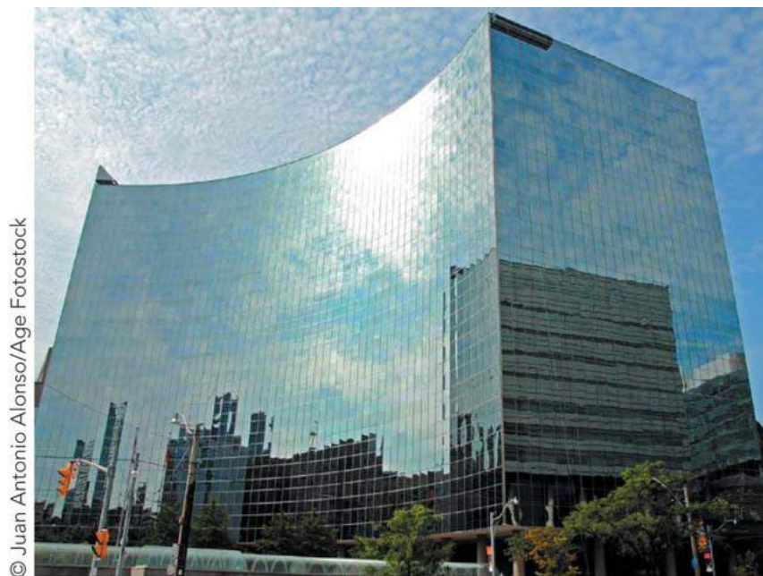
(b) A superinsulated office building in Toronto, Canada, has south-facing windows with insulating glass. The building is so well insulated it uses no furnace.
