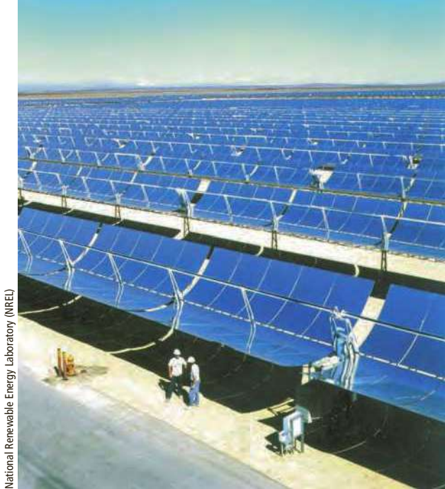
FIGURE 16.11 Solar thermal power: This solar power plant in California's Mojave Desert uses curved (parabolic) solar collectors to concentrate solar energy to provide enough heat to boil water and produce steam for generating electricity.
