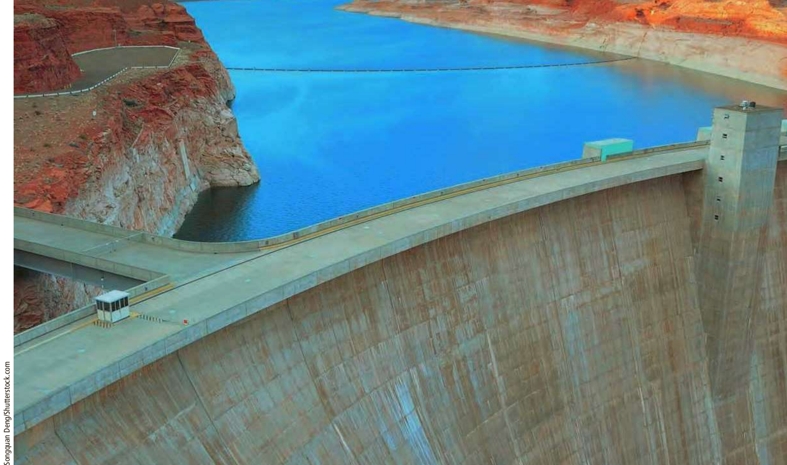
FIGURE 2.13 The water stored in this reservoir behind a dam has potential energy, which becomes kinetic energy when the water flows through channels built into the dam where it spins a turbine and produces electricity—another form of kinetic energy.
