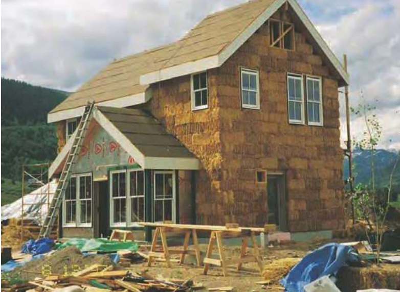
FIGURE 16.6 Solutions: Energy-efficient, Victorian-style straw-bale house in Crested Butte, Colorado, during construction (left) and after it was completed (right). Question: Would you like to live in such a house? Explain.
