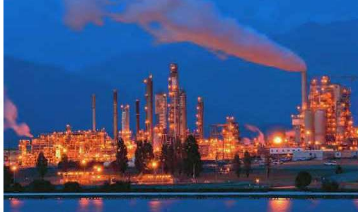
FIGURE 15.4 When crude oil is refined, many of its components are removed at various levels of a distillation column, depending on their boiling points. The most volatile components with the lowest boiling points are removed at the top of the column, which can be as tall as a nine-story building. The photo shows an oil refinery in Texas.
