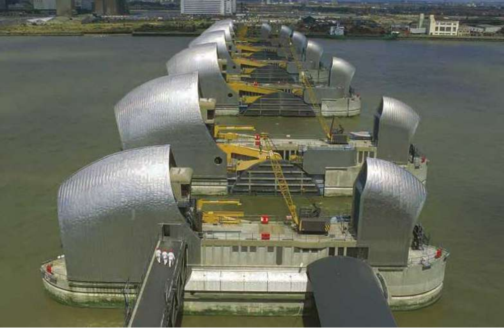
FIGURE 19.24 This high-tech, movable flood-control barrier—the second largest in the world—was built across the Thames River to prevent flooding from very high tides and storm surges in London, England.
