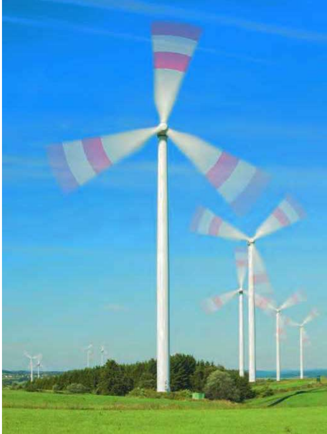
FIGURE 2.11 Kinetic energy, created by the gaseous molecules in a mass of moving air, turns the blades of these wind turbines. The turbines then convert this kinetic energy to electrical energy, which is another form of kinetic energy.
