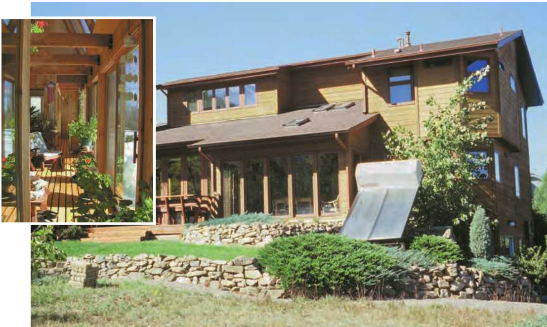
FIGURE 16.9 This passive solar home (right) in Golden, Colorado, collects and stores incoming solar energy to provide much of its heat in a climate with cold winters. Notice the solar hot water heating panels in the yard. Some passive solar houses have sunrooms (see inset photo) to help collect incoming solar energy.
