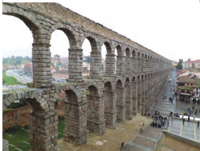
Figure 21.3 With the development of cities, humans began to interact intensively with the landscape at larger scales. This 2,000-year-old Roman aqueduct in Segovia, Spain, once transported water 18 km to the center of the Roman town. lovelypeace/123RF
