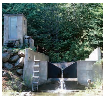
(a) Hubbard Brook dam and weir
