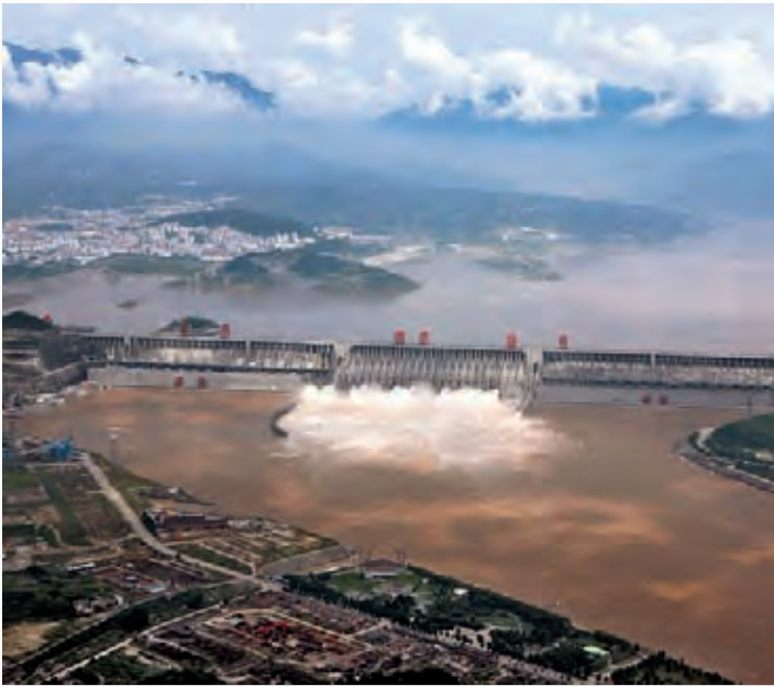
Figure 27.15 The Three Gorges Dam on the Yangtze River, China.
